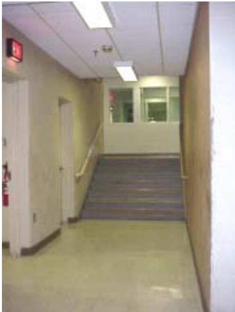
Figure 11 Access path to Medical Unit
