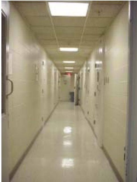
Figure 11 Housing Unit Corridor
