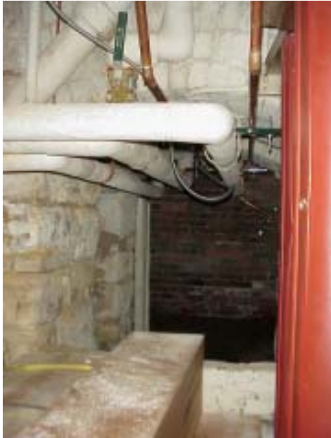
Figure 11 Mechanical Systems in Old Jail
