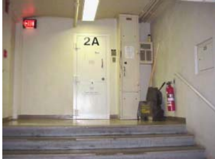
Figure 11 View of entry to Housing Unit 2A
