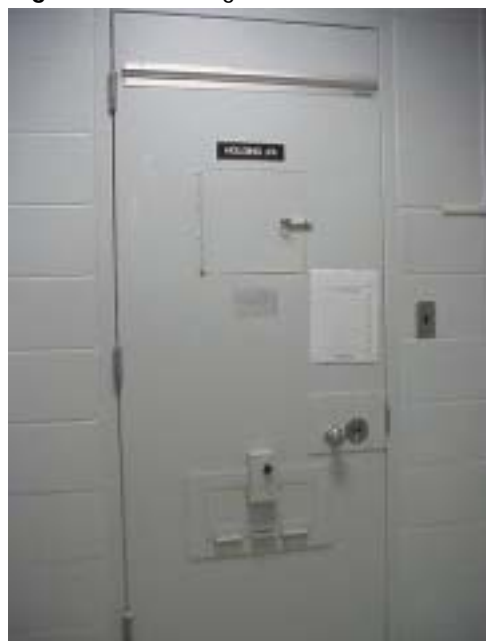
Figure 11 Holding Cell Door
